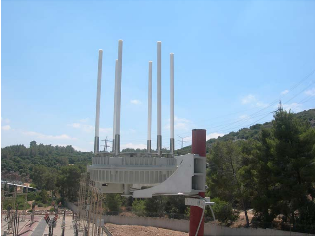
Figure 3.3 Mounting on a Metal Pole
