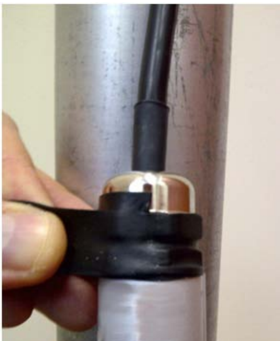
Figure 4-50: Protecting the unit joints with vinyl tape
