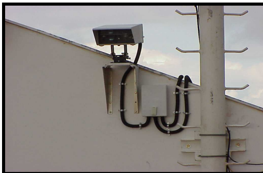
Figure 2.8: Wall Mounting (using JMP and JMB)
