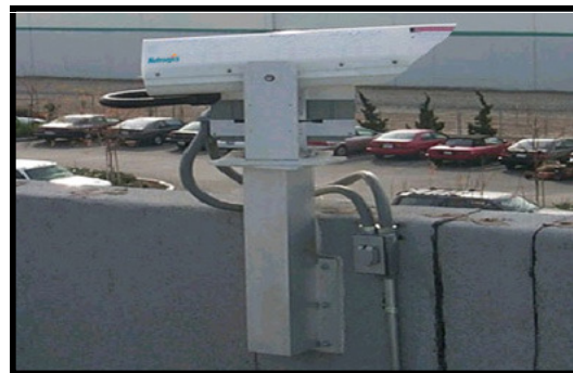
Figure 2.9: Wall Pedestal Mounting (using JMP & M054C)
