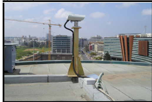
Figure 2.7: Floor Pedestal Mounting (using JMP and M015C)
