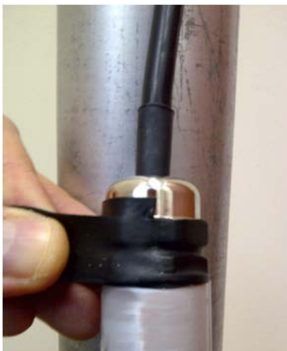
Figure 3-34: Protecting the unit joints with vinyl tape
